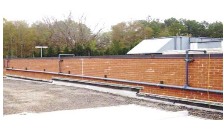
The collection manifold from each of the three units as the condensate is collected together. Image: EPA
